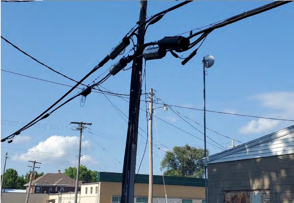
Fixed wireless CPE on a mast for Line of Sight to the Access Point (Auburn)
