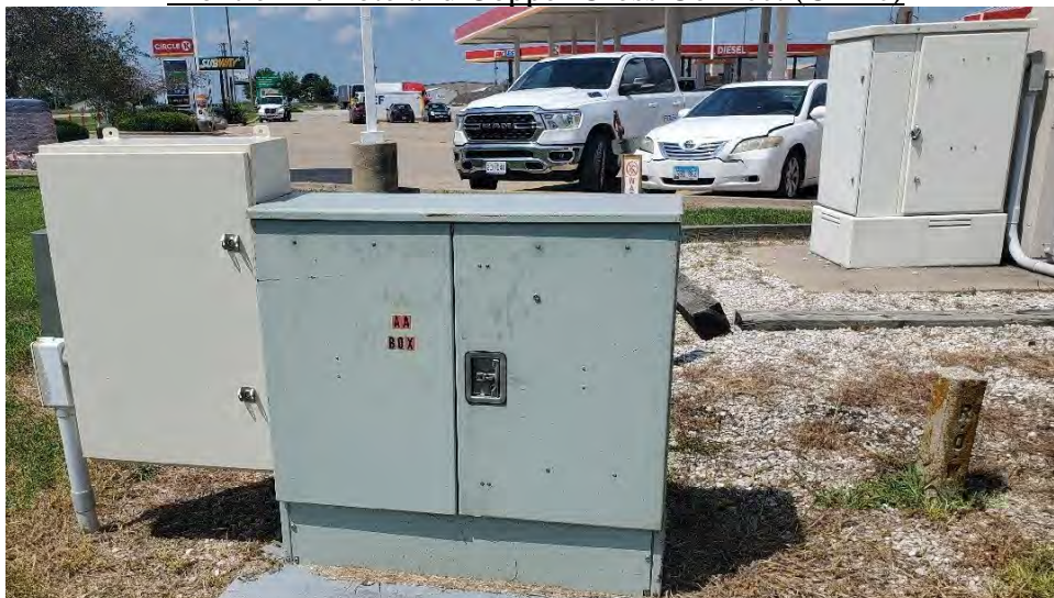
Frontier Remote and Copper Cross Connect (Cimic)
