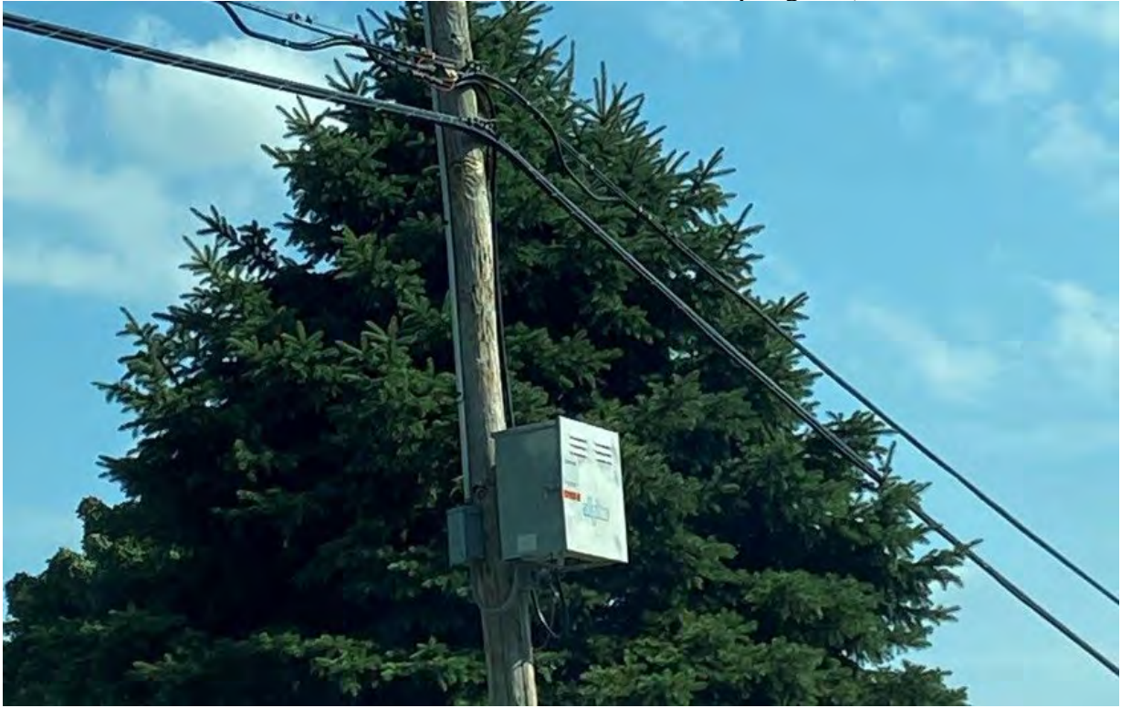
Comcast cable node (Rural area SW of Springfield)
